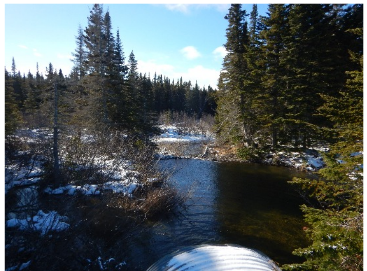
Ponceau Lac Rond / Culvert near Lac Rond
